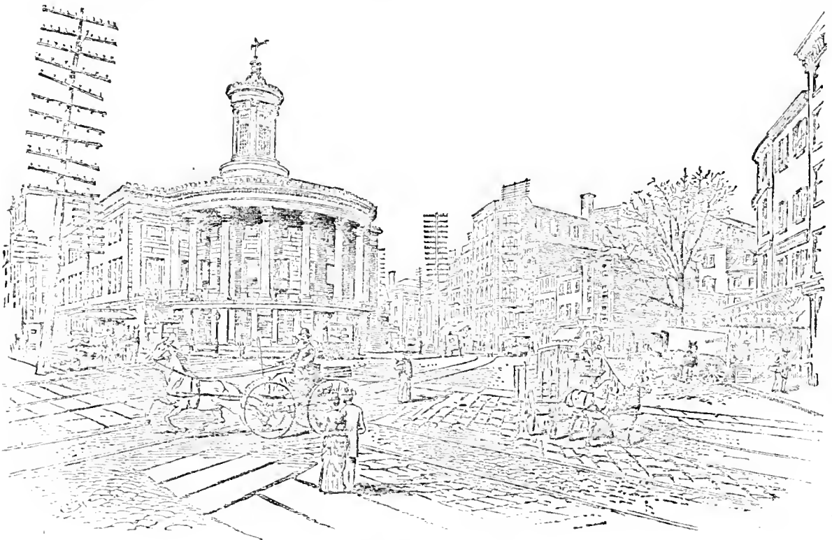
Dock Street, from Walnut Street.
